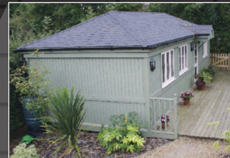
Accommodation Lodge by Homelodge Buildings
